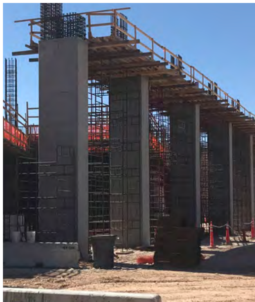
Column work continues on the South end of the Stadium.
