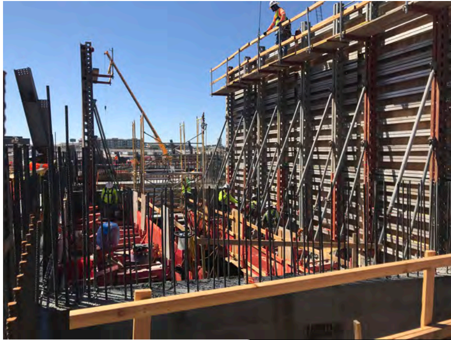
Work on the interior of Core #4.
